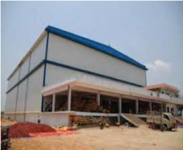
Fig. 1.8(a): Cold Storage
