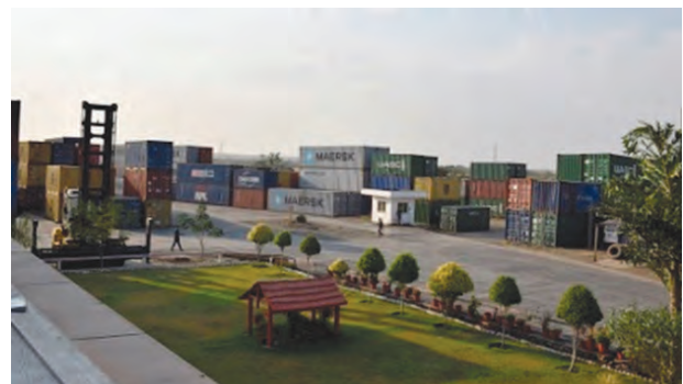
Fig. 1.11(b): Inland Container Depot
