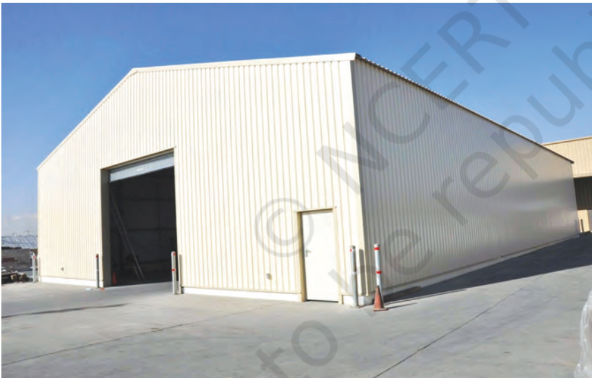
Fig. 1.25: A Portable Warehouse
