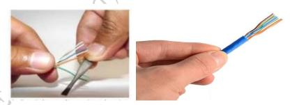
1. Straighten the twisted pairs 1. Arrange the wires in a row Fig. 2.12: Straightening and arranging the wires
