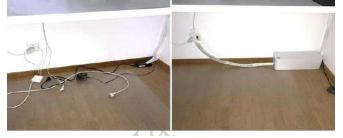
Fig.3.7: Safe and unsafe power cable arrangement
