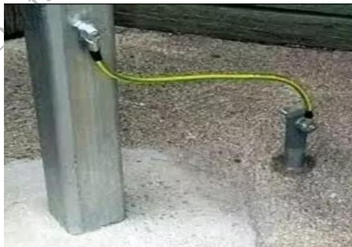
Fig. 3.45 Pipe Earthing
