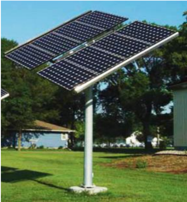
Fig. 2.21 Pole Mounting Structure
