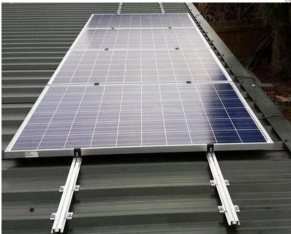
Fig. 2.13 Railed Mounting System
