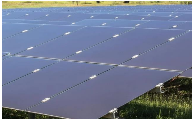
Fig. 2.10 Thin Film PV (Amorphous) Panels
