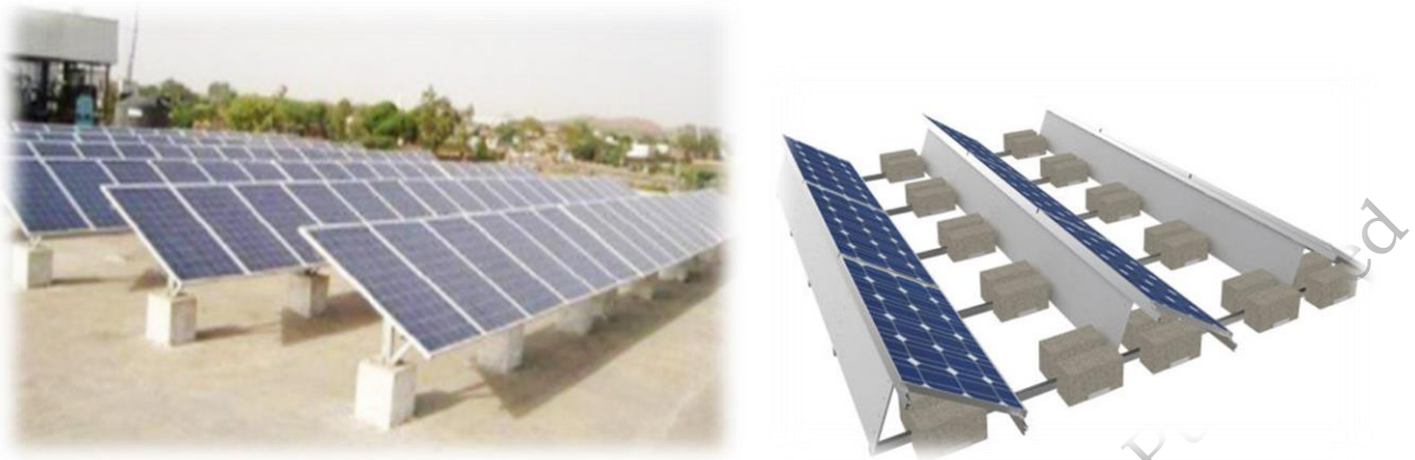
Fig. 2.14 Ballasted Mounting System
