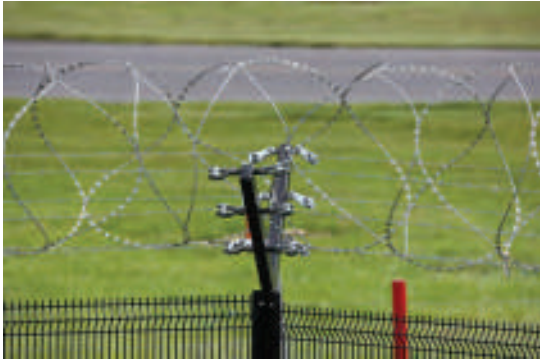
Fig. 4.6: Barbed wire and electric fence
