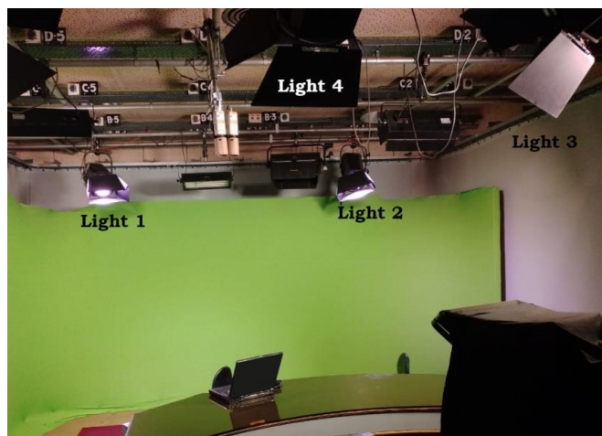
Fig. 2.14 Lighting setup for chroma key
