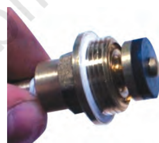
Fig. 6.8: Replacing the rubber washer
