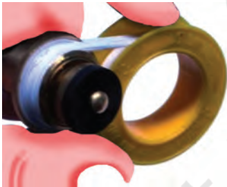
Fig. 6.9: Applying tape
