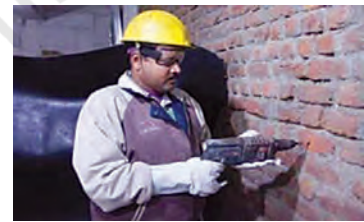
Fig. 6.1: Using power drill machine
