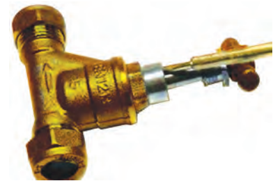
Fig. 5.4: Removing bits from a gland nut
