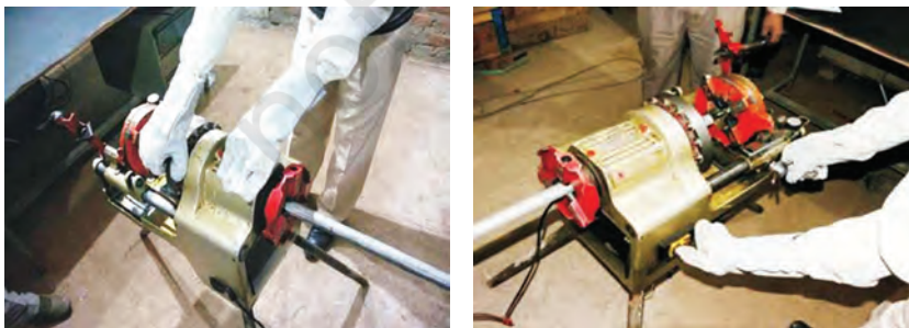
Fig.1.8: Pipe threading using pipe threading machine
