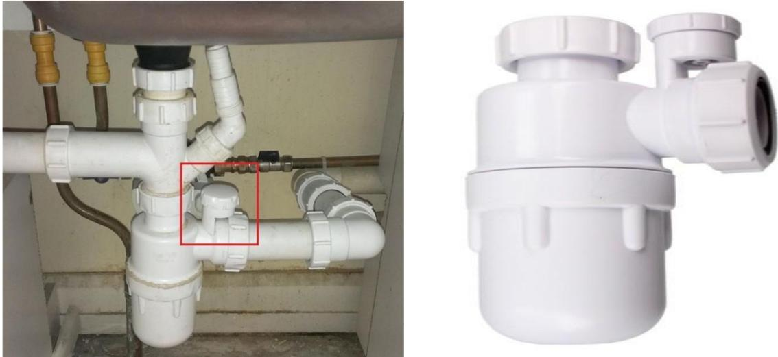
Fig 5.9 Anti-syphon Trap
