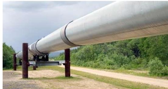
Fig 4.6 Over-Ground Piping
