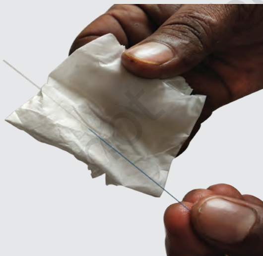
Fig. 5.20: Cleaning the jelly with dry tissue
