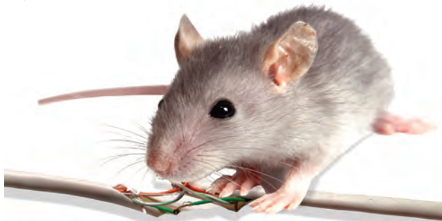
Fig. 5.3: Damage in fiber cable due to rodents
