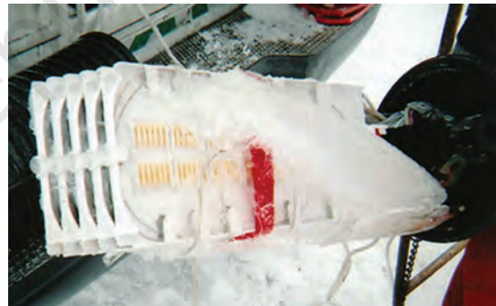
Fig. 5.6: Damage to the fibre cable due to ice crush
