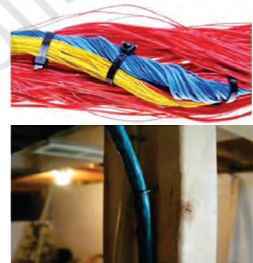
Fig. 9.75 Securing of cables
