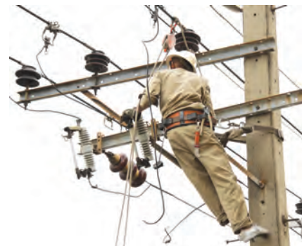
Fig. 1.1(b) A lineman repairing electric fault
