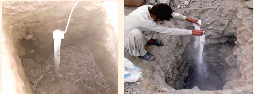
Fig. 4 Pit filled with mud, sand and stones
