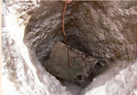
Fig. 2 Copper plate set in the pit
