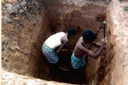
Fig.1 Making a pit for earthing
