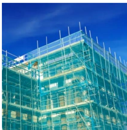
Fig.: 1.31: Scaffolding Nets
