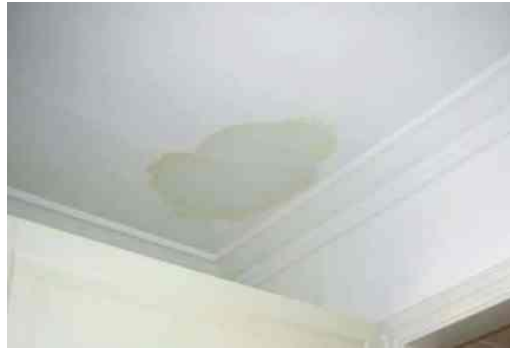
Fig 3.14 Blooming defect
