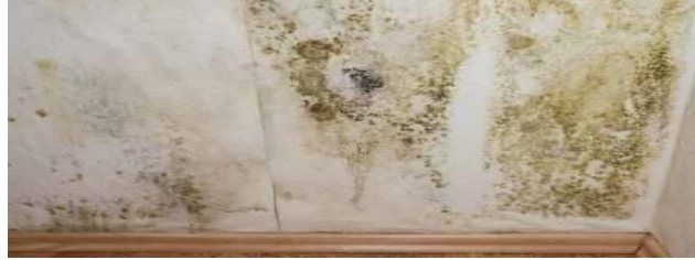
Fig 3.17 Mildew defect
