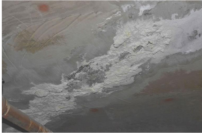
Fig 3.6 Efflorescence defect
