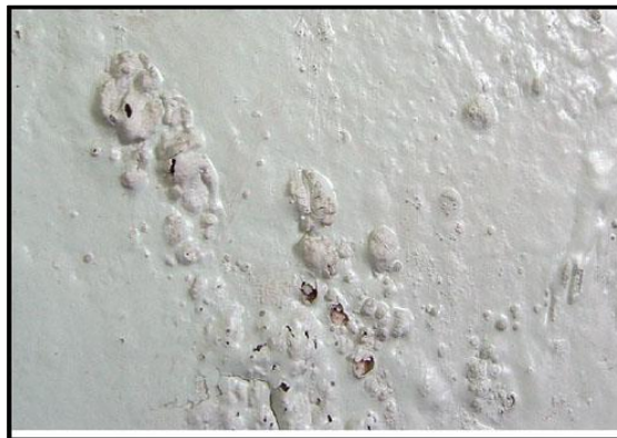
Fig 3.7 Popping defect
