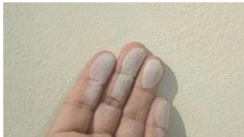
Fig 3.10 Chalking defect
