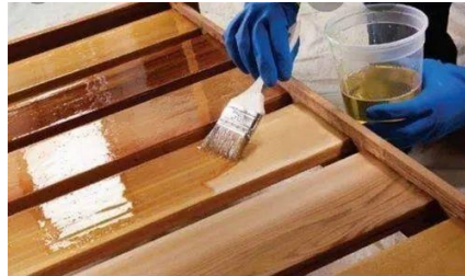
Fig 4.2 Applying varnish over wooden surface
