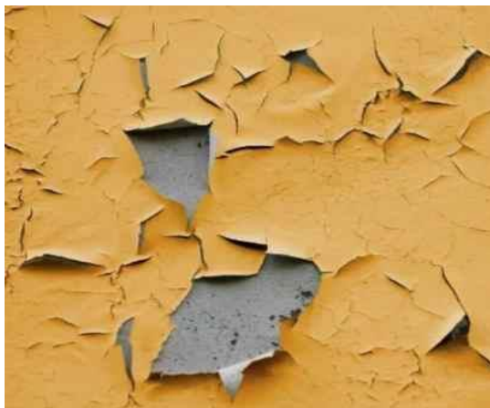
Fig 3.13 Flaking defect
