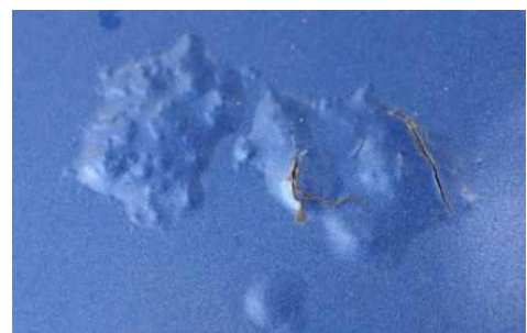
Fig 3.8 Blistering and Peeling
