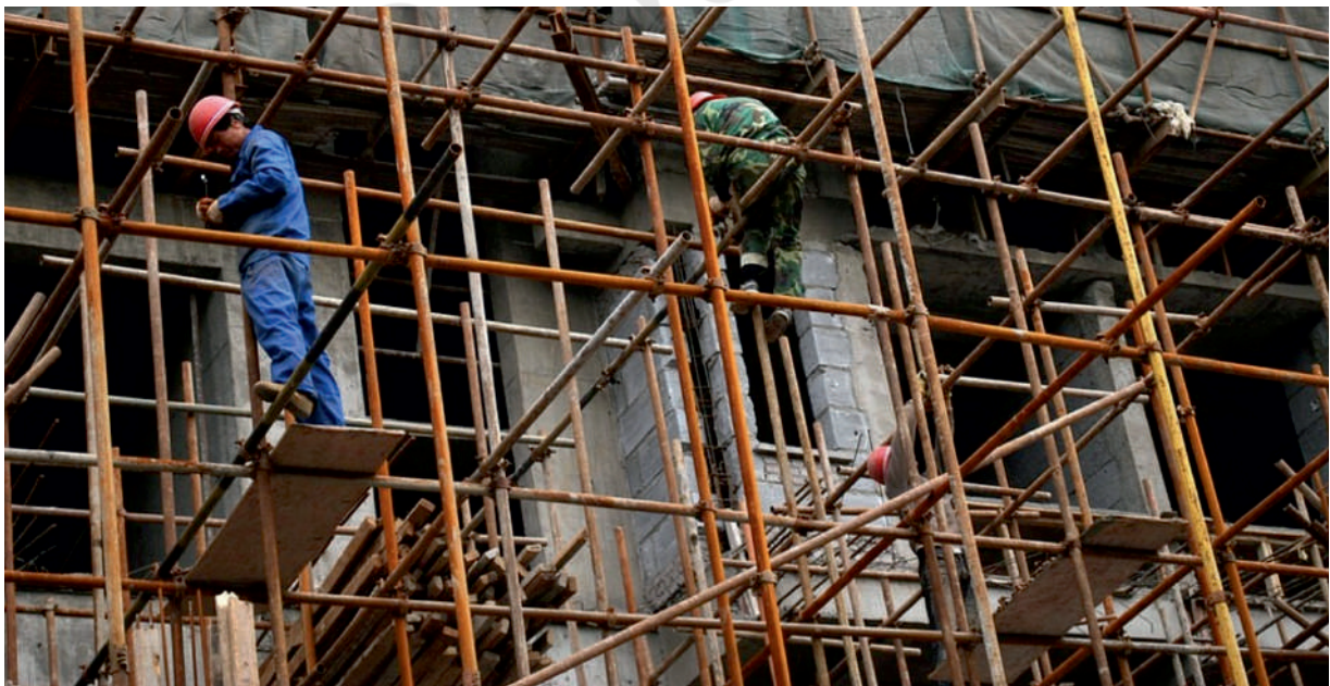
Fig. 3.1: A view of Scaffolding
