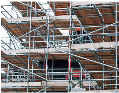
Fig. 3.7: Cantilever Scaffolding
