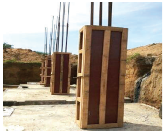
Fig. 4.3: Formwork for square or rectangle columns
