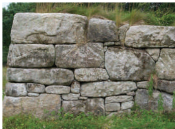
Fig. 1.11: Dry rubble masonry
