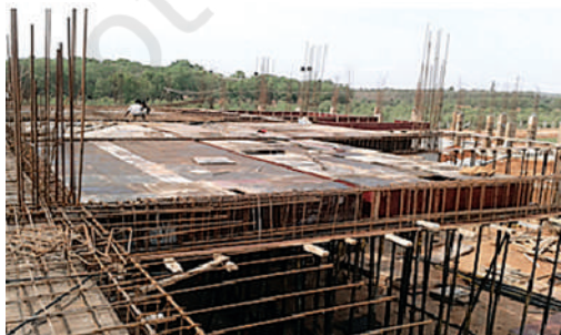
Fig. 4.4 (a): Shuttering for beam and RCC Floor
