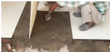
Step 2: Pasting of mortar
