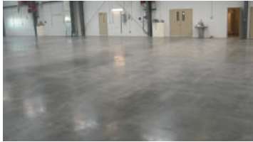
Fig. 5.4: Cement concrete flooring
