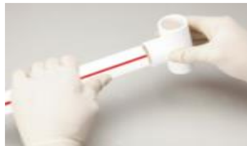
Fig.3.8: Fitting preparation of pipe
