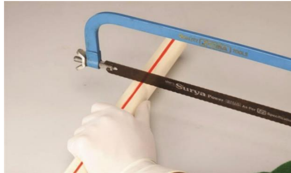
Fig.3.6: Cutting the pipe
