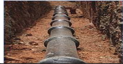
Fig.3.19: Laying of Stone ware pipe
