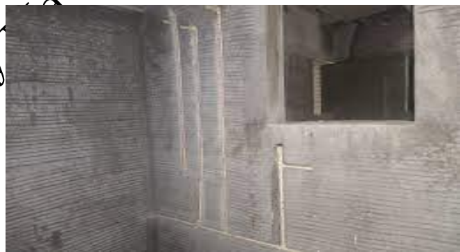
Fig.3.57: Concealing of pvc pipe inside the wall
