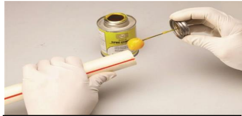
Fig.3.9: Solvent application of pipe
