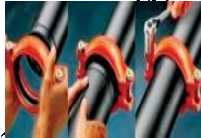
Fig.2.36: Grooved Joint
